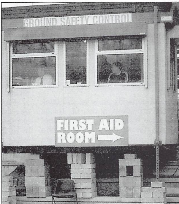
MARK FAWCETT The Shay safety control box . . . "propped up on breeze blocks".
