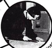
Wood Work & Joinery
