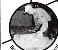
Brick Work & Construction
