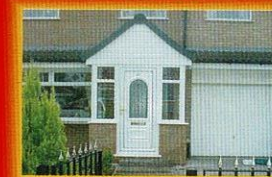
Replaced or built from scratch
