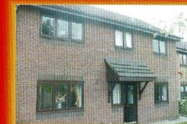
PVC Door & window canopies supplied and fitted
