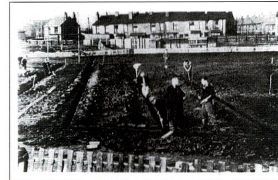
February 1947 - Tommy Sale (Foreground, Right) discussing the laying of the new drains at the Charles Street ground with Leigh manager Fred Pemberton.
